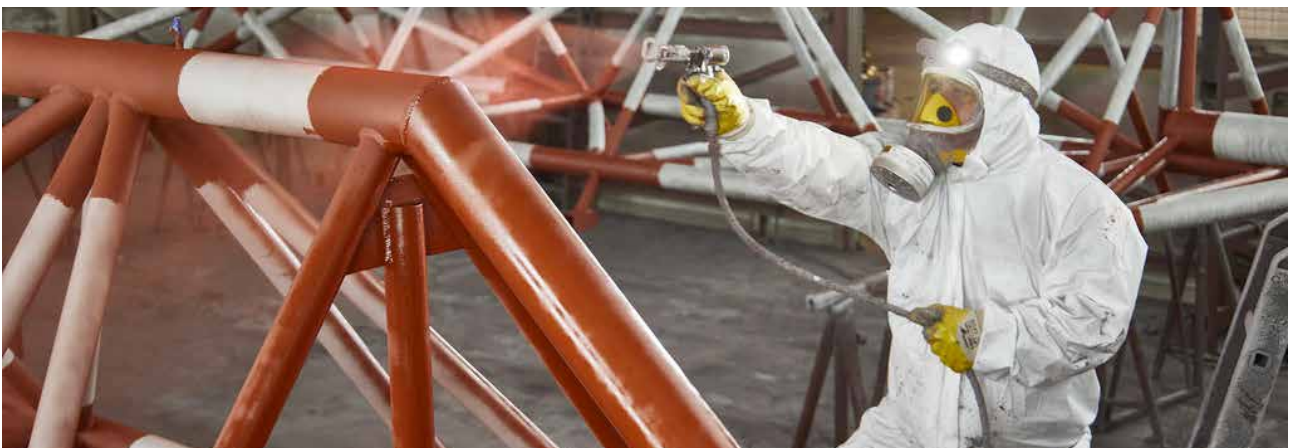
Application of surface protection
