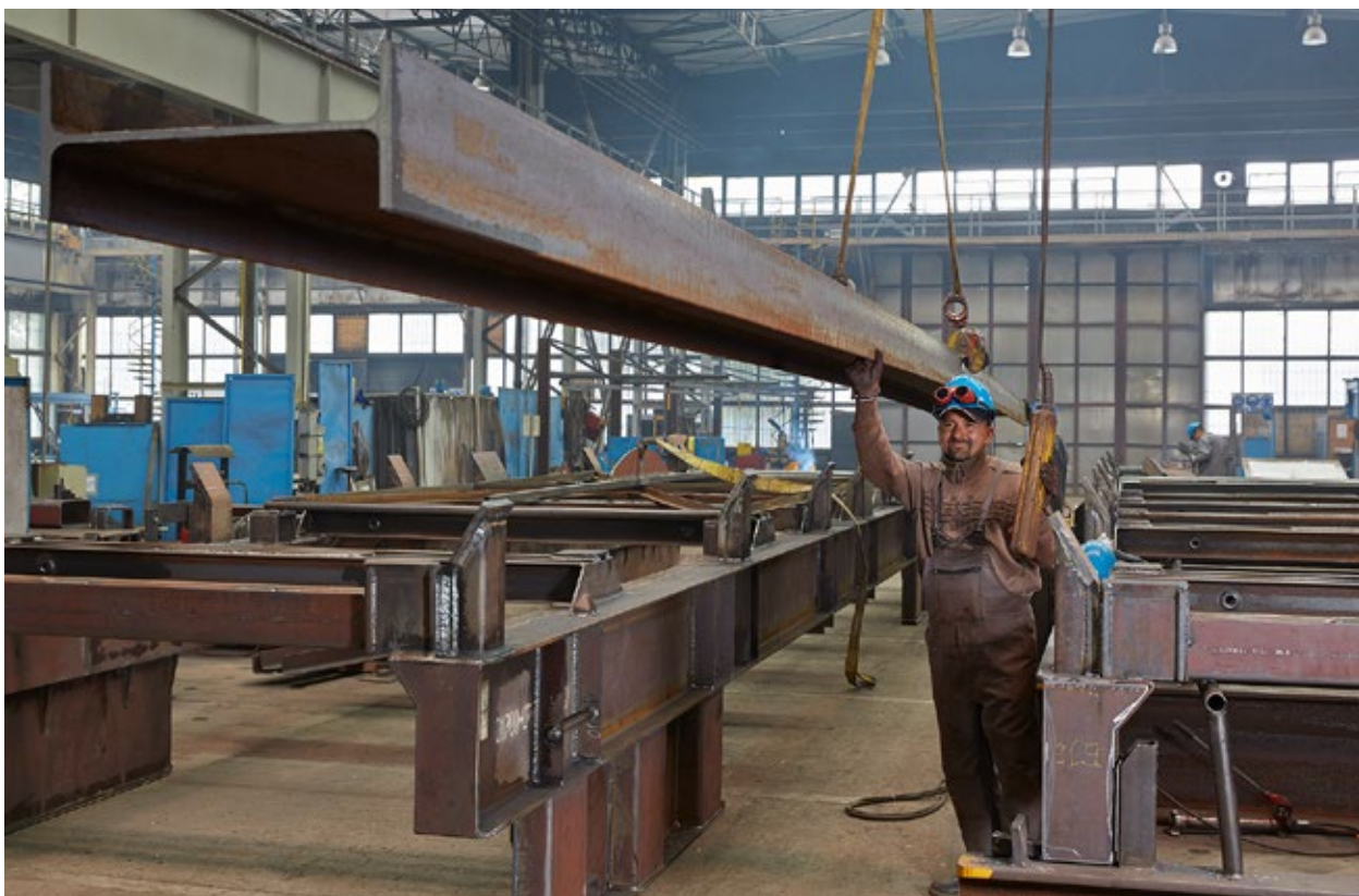
Steel construction in Szczecin, Poland
