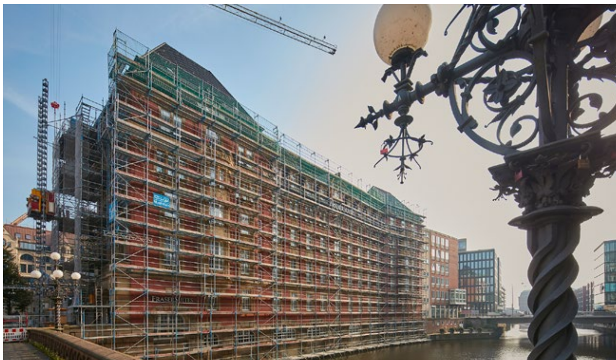
Scaffolding in Hamburg, Germany
