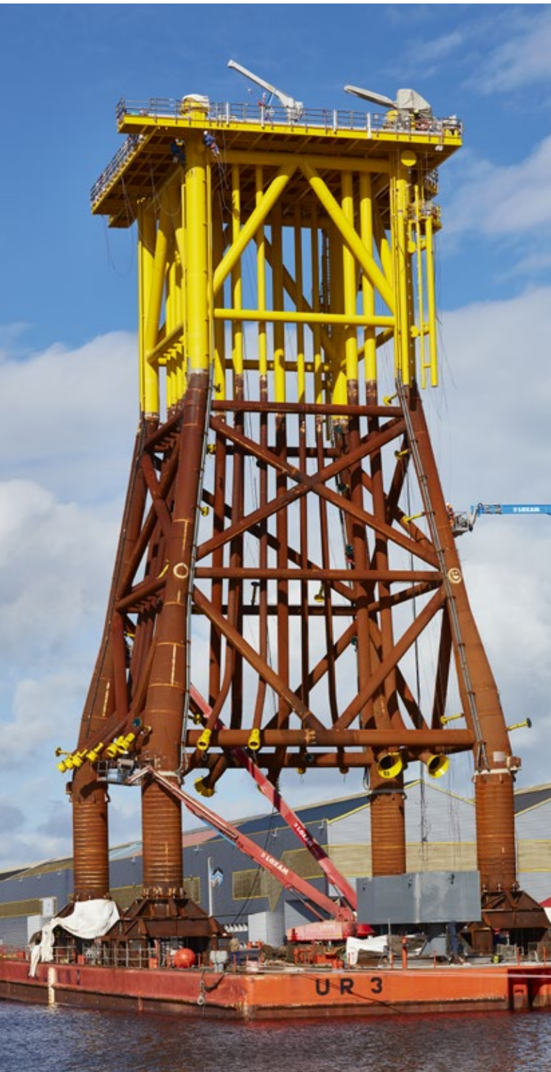
Jacket construction for offshore wind power station in Saint-Nazaire, France
