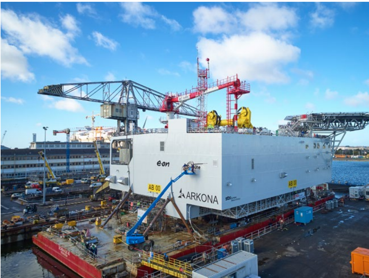
Offshore transformer platform in Saint-Nazaire, France
